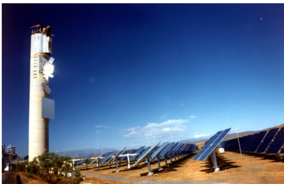
Figure 4: Experimental central receiver system at the European research center Plataforma Solar de Almería in Spain
