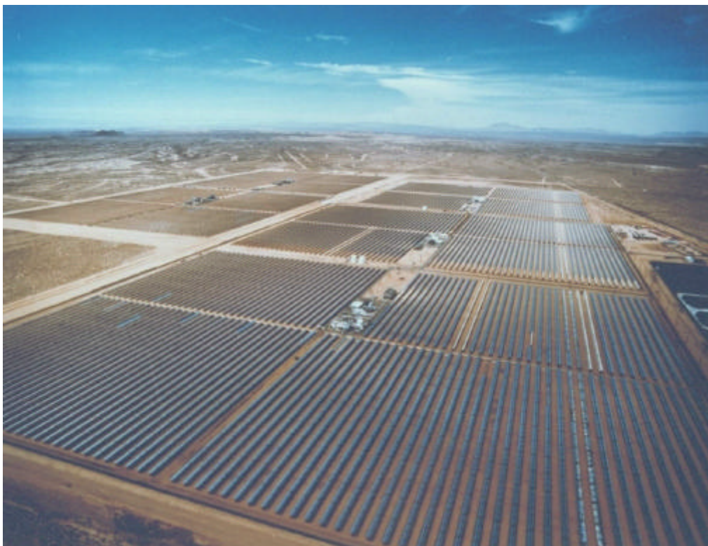
Figure 5: Aerial view of the solar thermal power plants at Kramer Junction in the US-Californian Mojave desert (photograph: KJC)
