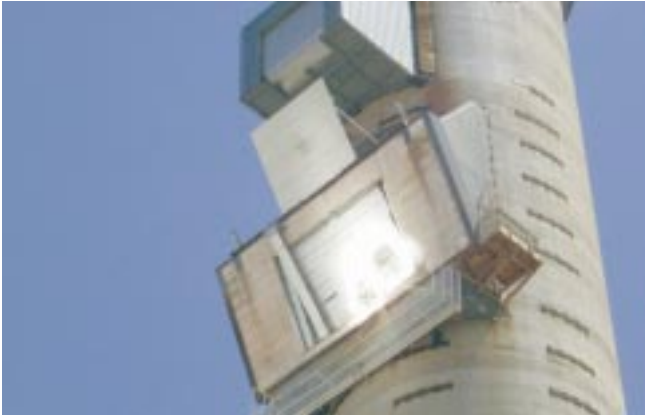
R&D leading to efficiency improvement in the volumetric receiver (above) will be supported.
