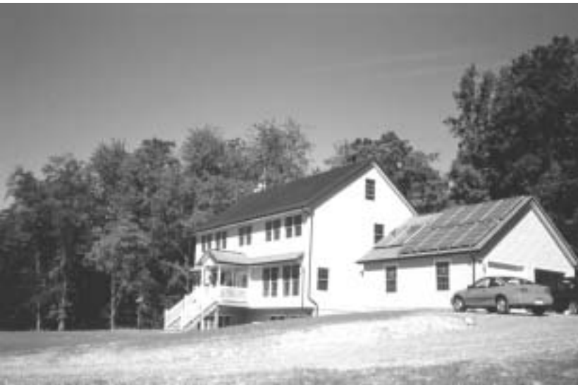
The Solar Patriot was recently "installed" in Purcellville, Virginia. The house is modular in construction and includes 6 kilowatts of PV modules, a solar water-heating system, an upgraded building envelope, and low-emissivity (low-e) windows. It will consume about 50% of the energy of a conventional home. The Solar Patriot was developed under the U.S. Department of Energy's Building America Program and was displayed on the National Mall in Washington, D.C. in April 2001.
