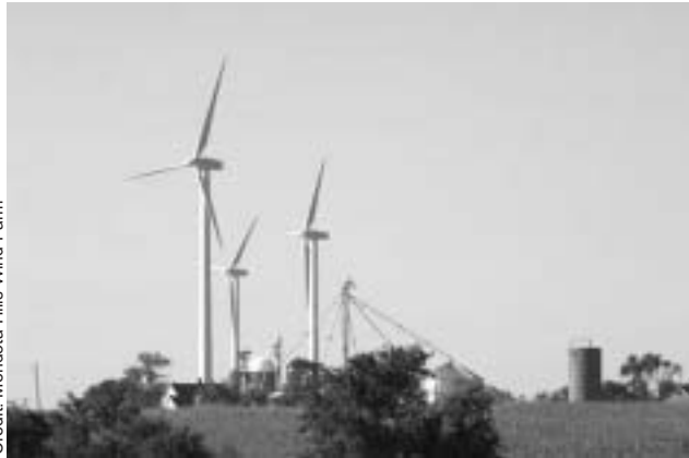
Credit: Mendota Hills Wind Farm
