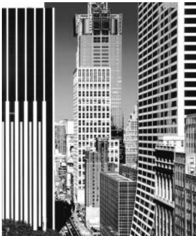
NREL/Andrew Gordon Photography and Fox & Fowle Architects
