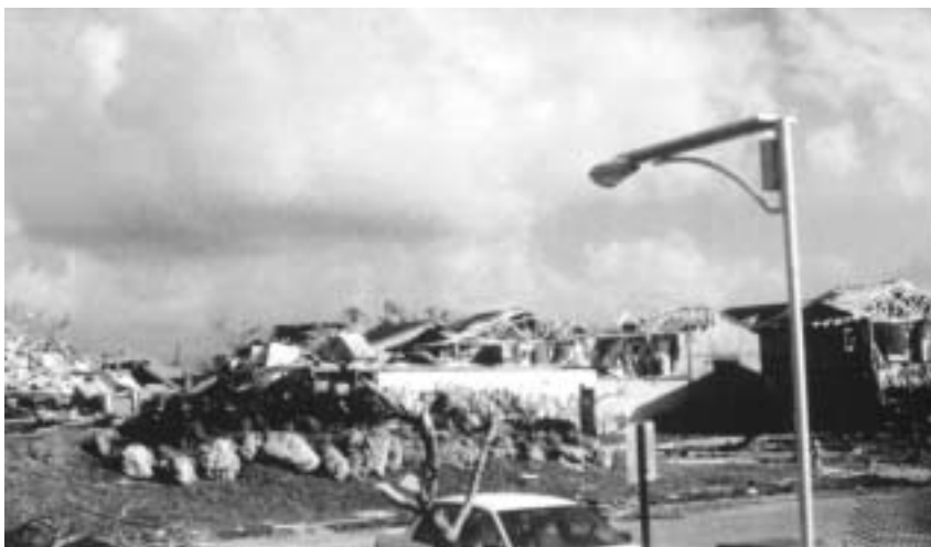
This suburban Miami street was lit by solar power after Hurricane Andrew struck in 1992. Solarpal safety streetlights not only survived Hurricane Andrew, but lit their communities until grid power was restarted 33 hours later.
