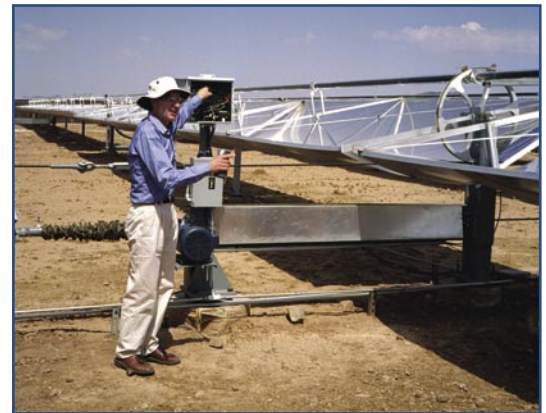
Parabolic trough concentrator modules at the Phoenix Federal Correctional Institution produce up to 50,000 gallons of hot water daily—enough hot water for kitchen, shower, laundry, and sanitation needs for 1,250 inmates and staff.
